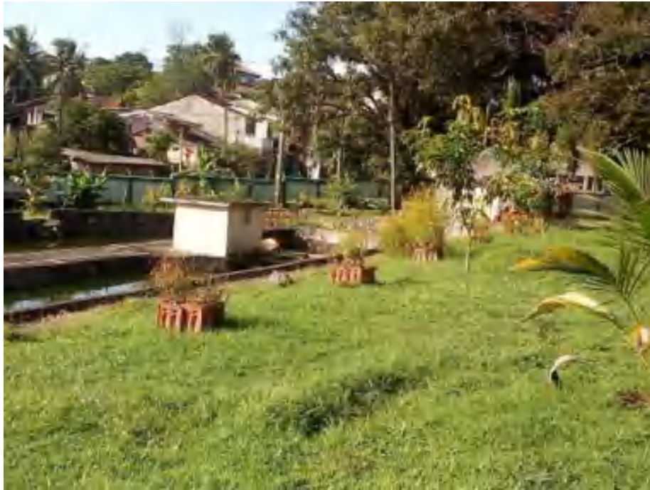
Existing sewerage plant
