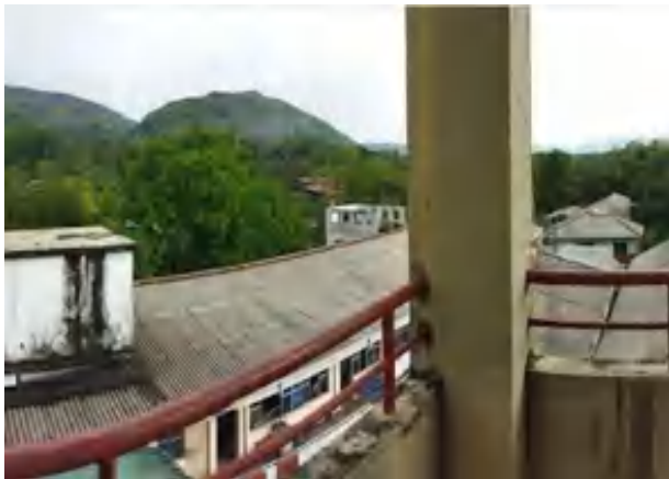
Asbestos roofing sheets at Karawanaella BH
