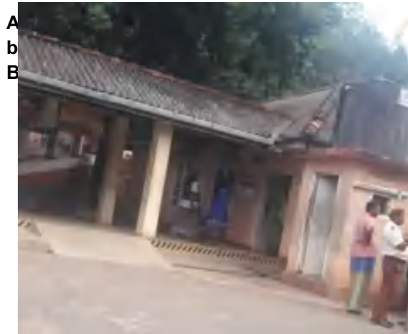
Asbestos roofing sheets & ceiling sheets to be removed during demolition at Kahawatta BH
