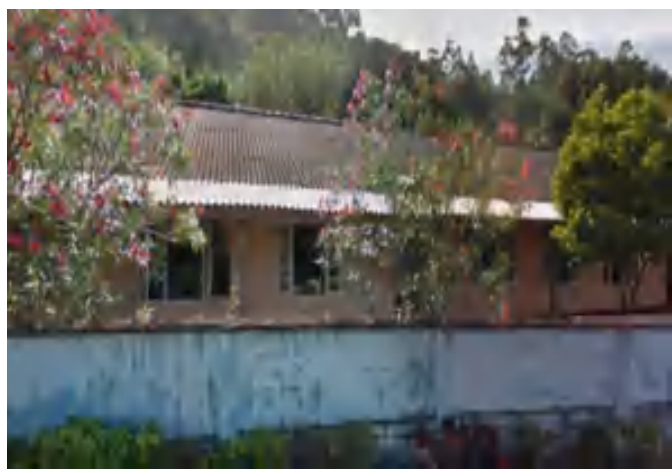
Asbestos roofing sheets & ceiling sheets to be removed during demolition at Kahawatta BH
