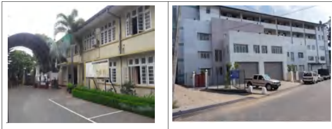
Figure 10. Photographs of Teldeniya BH
