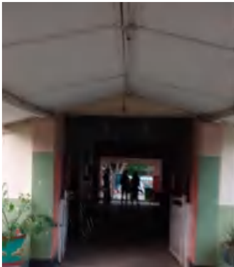
Asbestos roofing sheets at Karawanaella BH
